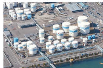
The Company’s Shiohama Teizan Oil Depot, a stockpiling and shipping base for next-generation biofuels
